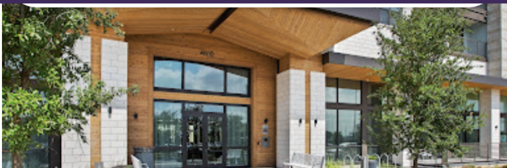
The Overture in Mueller — 4818 Berkman Dr, Austin, TX 78723
